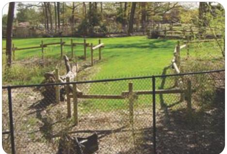
At left is another view of the giraffe restraint fence showing the chain link and post and rail portions. Above, elephants are restrained by this heavy-duty gate constructed of 6%-in. horizontal, diagonal and vertical rails, all coped and welded. The posts are 6-in. wide flange beams set 8-ft. into the ground, with the gate swinging on custom hinges. The gates are 8-ft. tall and 13-ft. wide. Below, a detail of a rhino/zebra swing gate.
